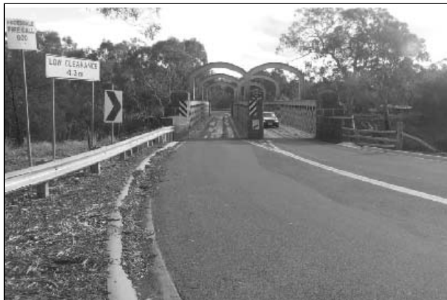
The iconic Campaspe River bridge on the Kyneton Heathcote Road.
